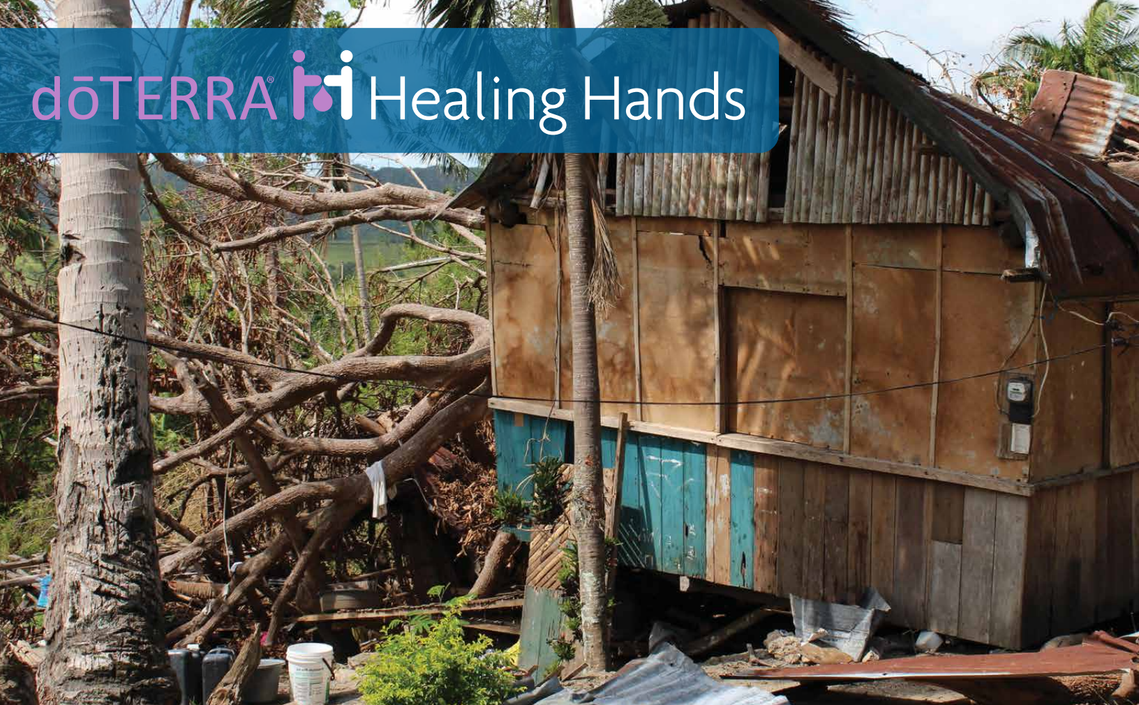
An example of damage caused by Typhoon Haiyan
